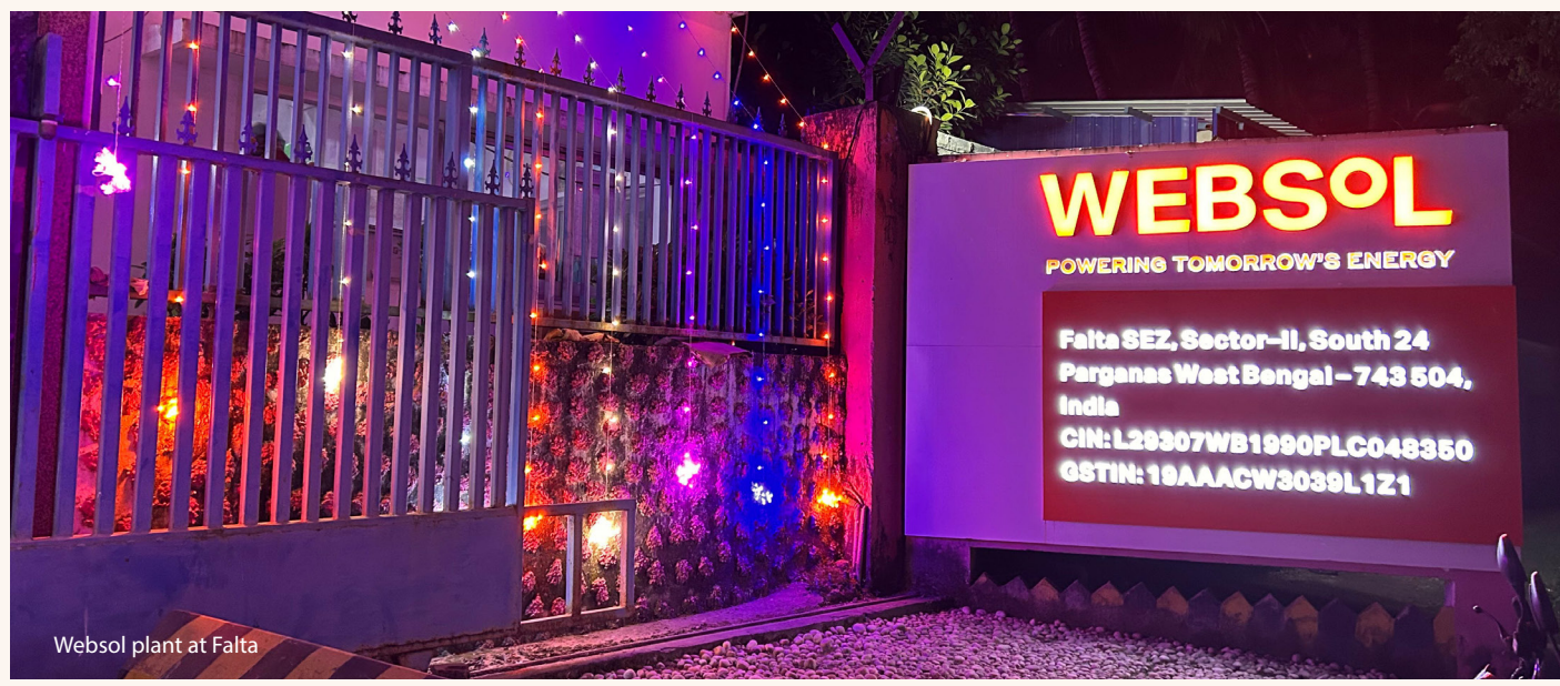
Websol plant at Falta
